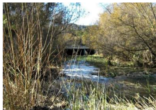
The City of Poway implements stormwater BMPs to manage surface water quality
